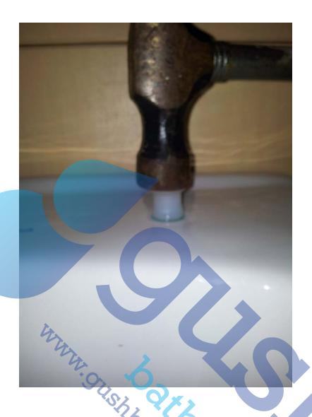
3). If brave you can use a standard hammer but remember one false slip will probably result in a broken pan. Using a rubber/plastic mallet can be of use but most people don't have one. The majority of us however have a metal hammer. Using a block of wood can add vital protection as pictured. You do have to use a fair bit of force but once it starts to ease in to place it will become easier.
