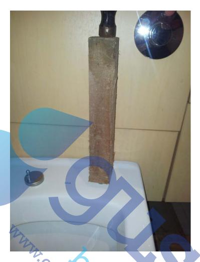
4). The last 2 pictures show the plug now installed and in place, then we can see the fitting of the hinge disks.
